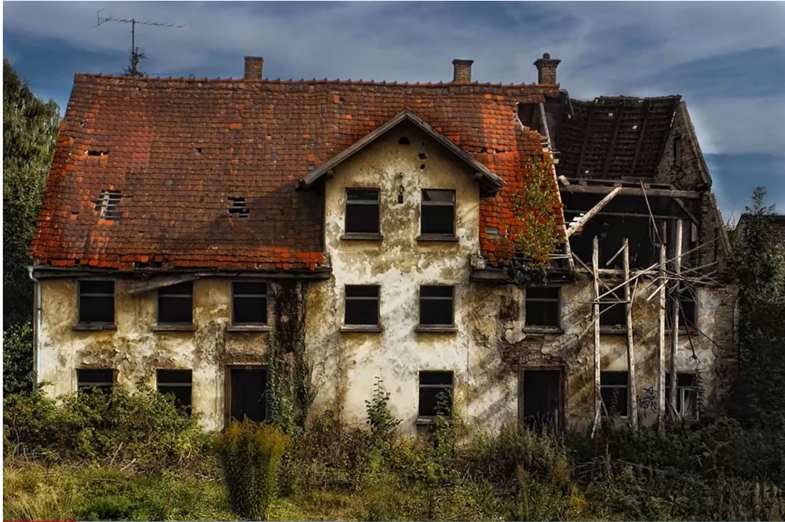
"ruined house" by pxhere is licensed under CC BY 4.0
